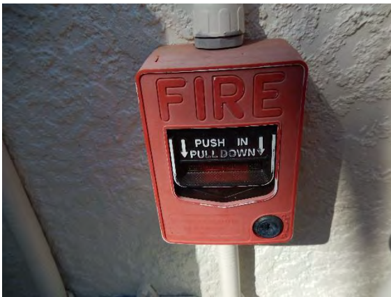
TYPICAL MANUAL FIRE ALARM
